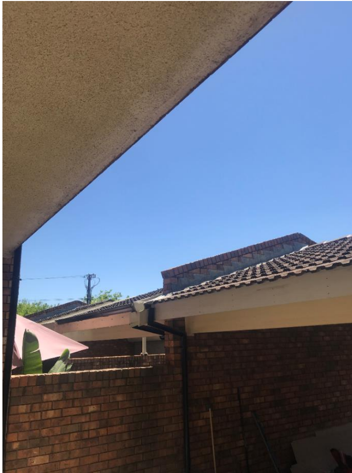
Figure 2 – Existing open space above existing masonry fence
