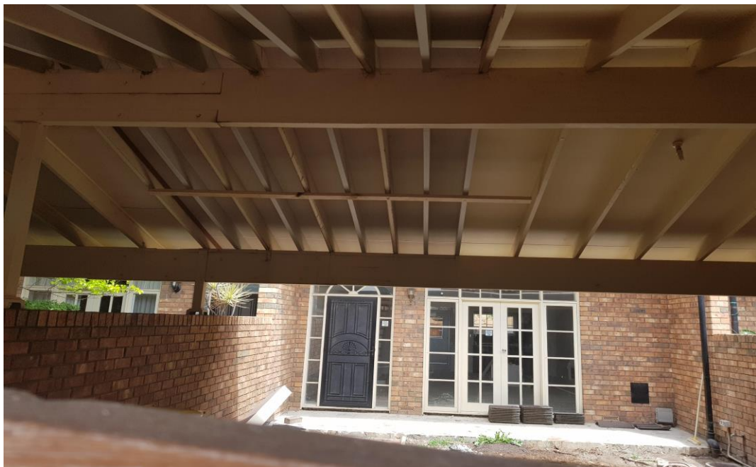
Figure 1 – Existing carport showing of raised roof construction
