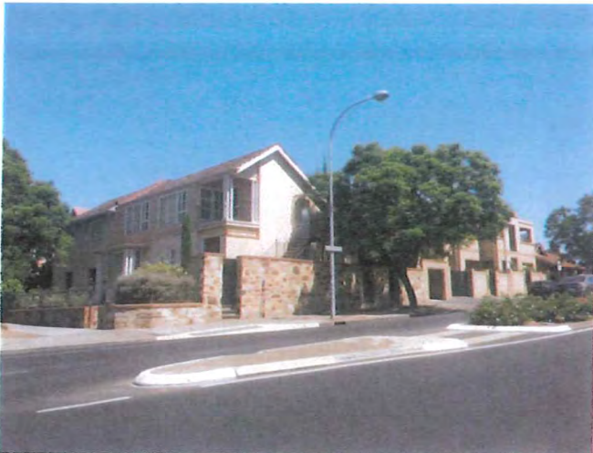
Overall view of the existing house from the SE showing two storey height character
