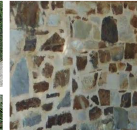
EXISTING BLUESTONE WALLING
